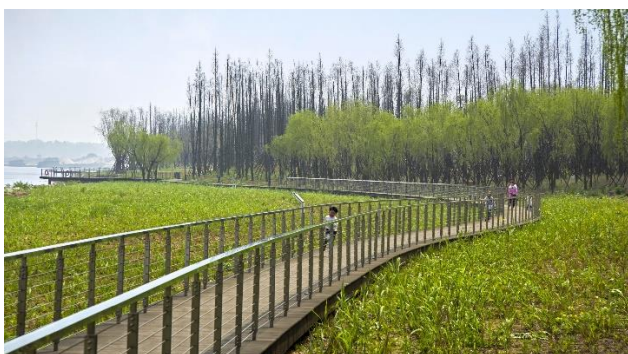
Trails and boardwalks lead the visitors through a meandering journey of discovery. Hidden surprises await in the forest, while commanding views define the wetland experience. Local condensed bamboo, a light-weight material resistant to flooding, is employed.
